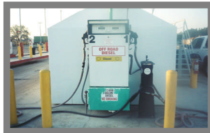
Model 2075 filtering on-road diesel and off-road diesel fuel for this customer. They are experiencing longer OEM filter life and fewer service calls related to dirty fuel.
